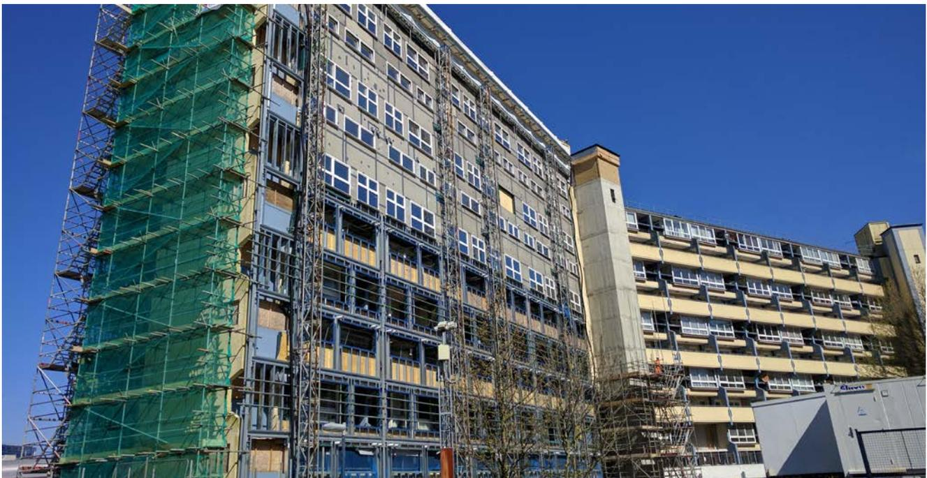
**Figure 6.14** - Courtyard side during construction, showing new EWI and triple-glazed windows being fitted. ECD Architects.
