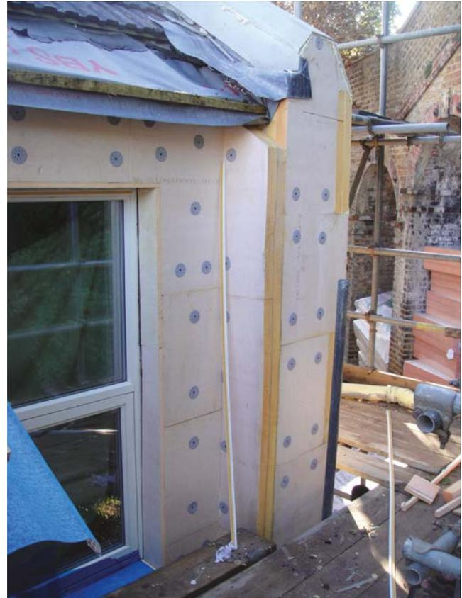
**Figure 6.12** - Installation of external wall insulation - BBM Sustainable Design
